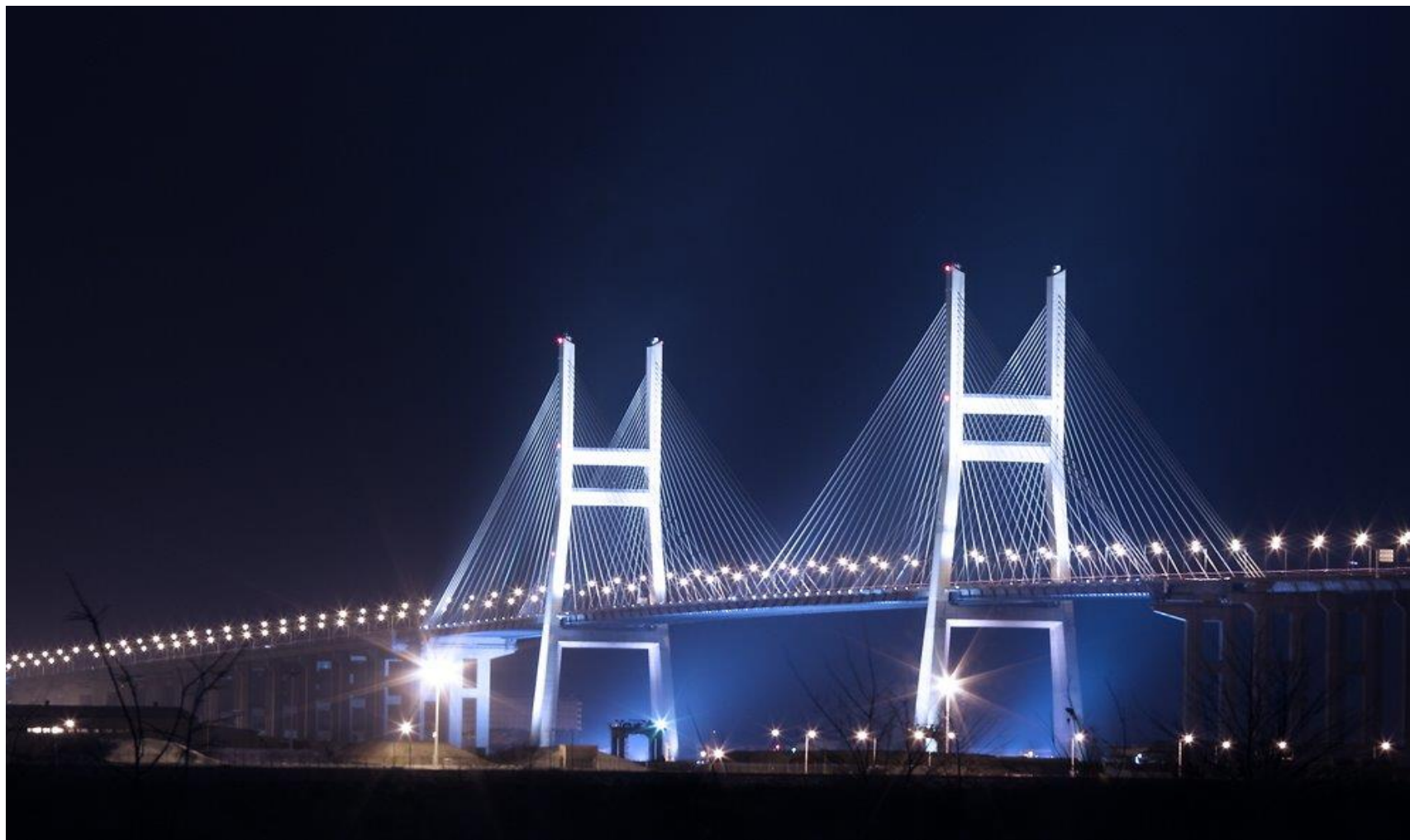
Seohae Grand Bridge in South Korea
