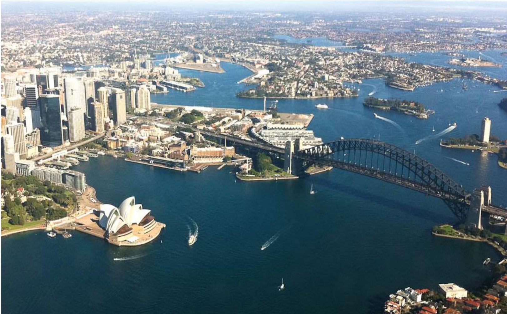
Australia – Sydney Harbor Tunnel
